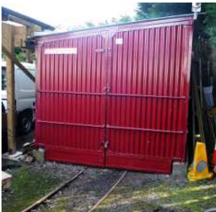
Newly painted engine shed
