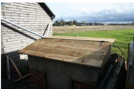
Coal bunker with new wooden top
