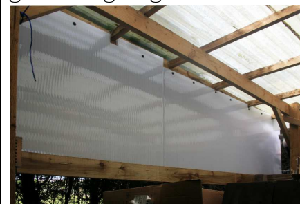
Fitted polycarbonate sheet at back of car port
