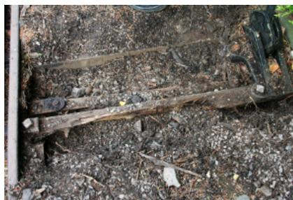
*The above photo shows the rotten wood between the rails on the point.*
