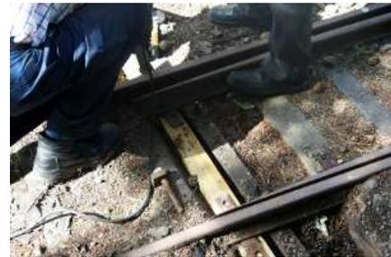
*The rotten wood has been removed and new wood (a fence post) has replaced it.*
