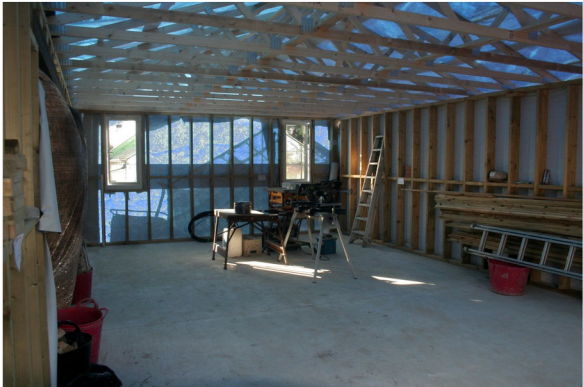
Before the roof went on
