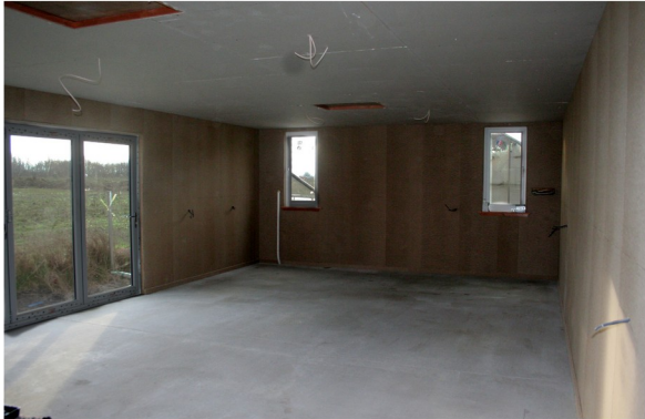
Roofing, lagging and walls fitted
