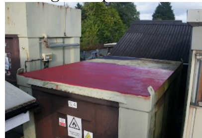
The newly painted roof on S4
