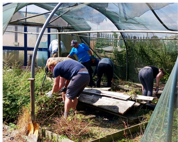
Clearing the shade tunnel
