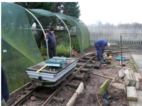
Setting out the curbs edges
