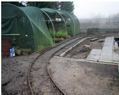
The job done
