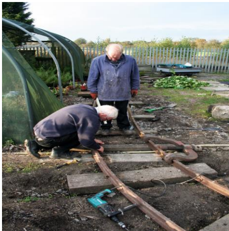
Using the Jim Crow to set the curve of the rail
