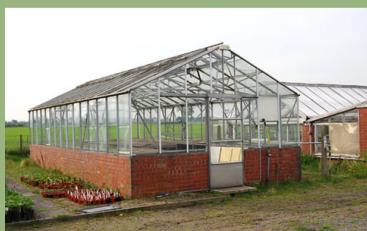
After having some panes of glass replaced Greenhouse G12 is now ready for use
