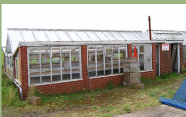
Greenhouse G7 & G8 A volunteer has power washed the glass panes removing moss and a build up of grime
