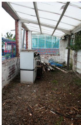
The space which will be covered by the car port-style roof.
