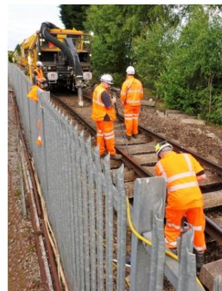
*Dayglo army removing ballast, it is sucked up by the machine in the background*
