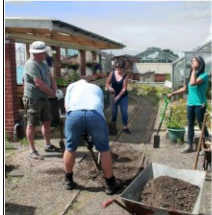
*Digging out the track to replace the sleeper*
