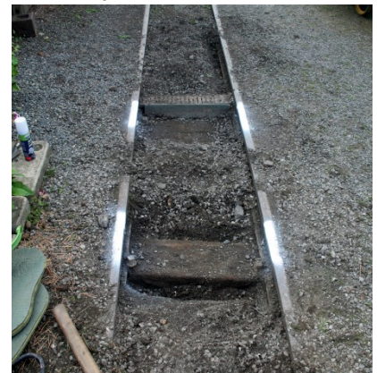
The excavated sleepers, the one furthest from the camera was replaced
